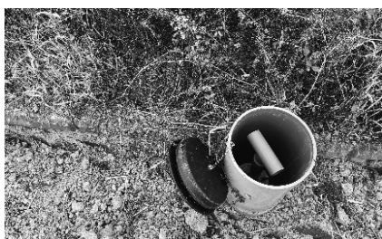
豎管式水閘暗渠
